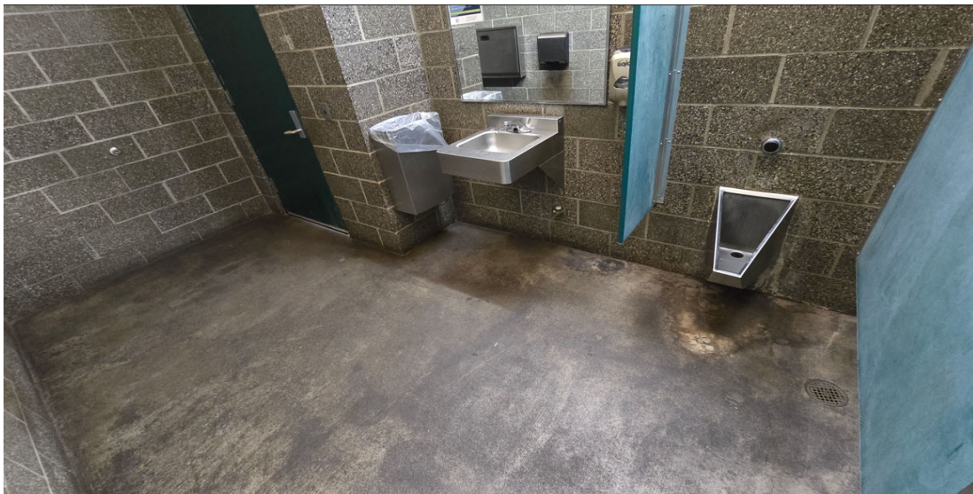
Reseal concrete floors at the Tualatin Hills Nature Center
