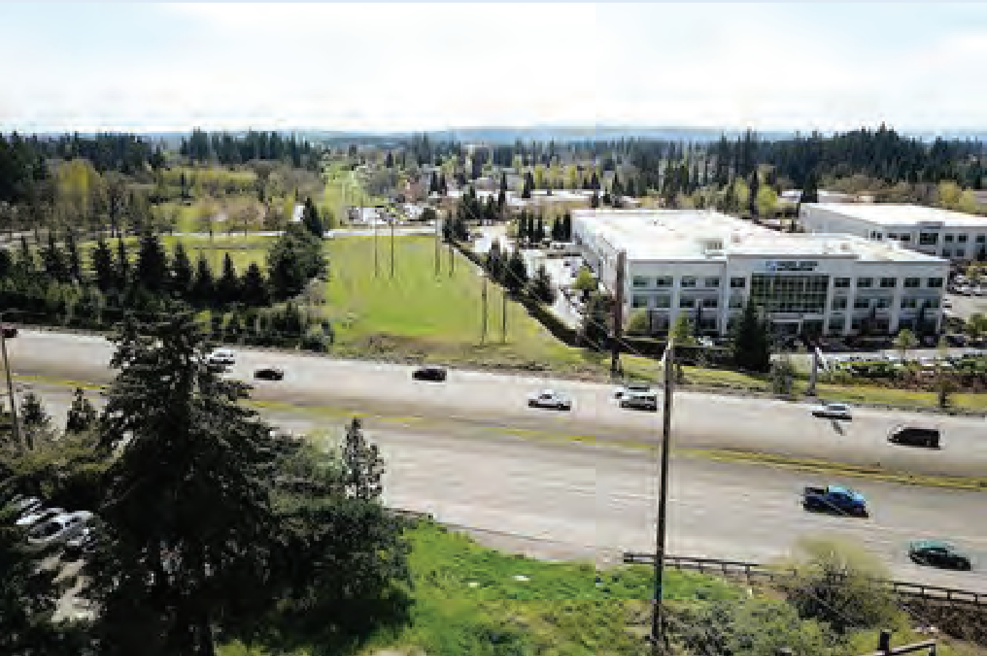
The grass area pictured above shows the location of the future Westside Trail Pedestrian and Bicycle Bridge.
