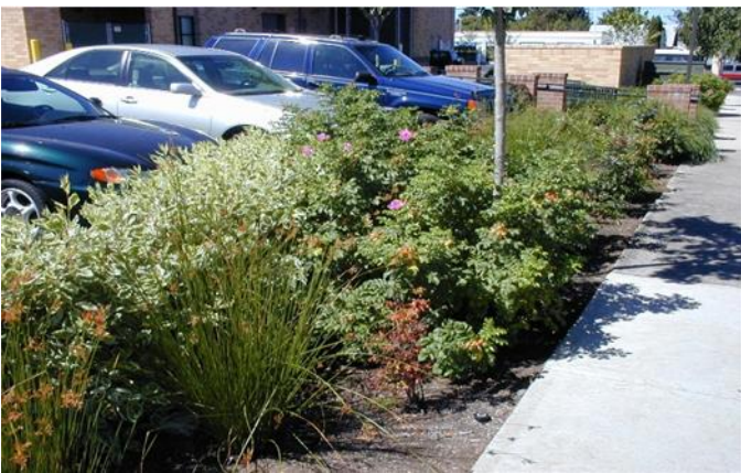
Figure 8. Vegetated Filter Strip (New Seasons 33rd Ave.)
