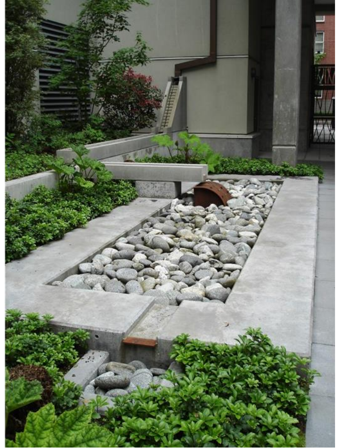
Figure 9. Stormwater Planters (Pearl District)
