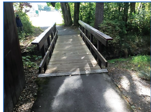
Hazeldale Park bridge before
