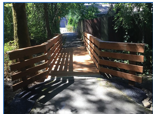
Hazeldale Park bridge after
