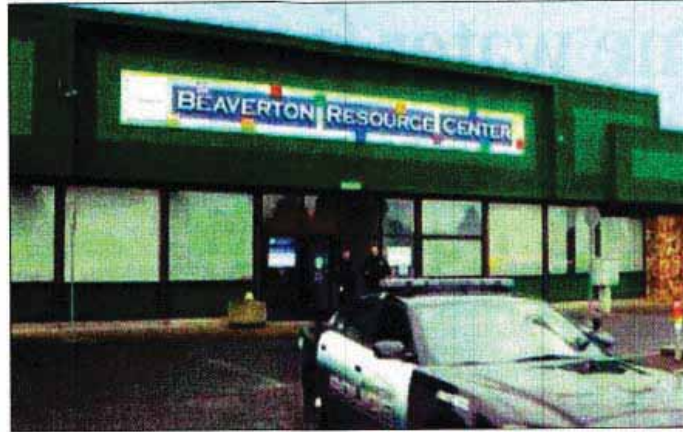
PAL will move its programs this fall to accommodate a new emergency services building. COURTESY: POLICE ACTIVITIES LEAGUE
